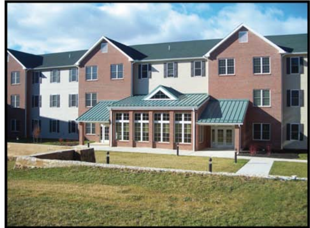
Newly constructed units at Hopewell Courtyard (January 2012).
