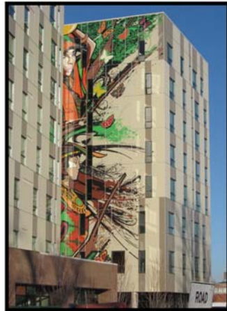
Newly constructed tower at 10th and Osage Senior/Disabled Housing and Community Center (December 2011), Denver Housing Authority.
