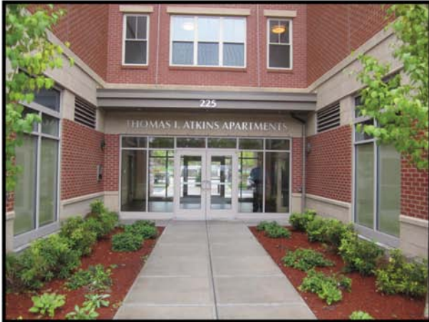
Newly constructed Thomas L. Atkins Apartments (September 2011), Kasanof Bakery Project.
