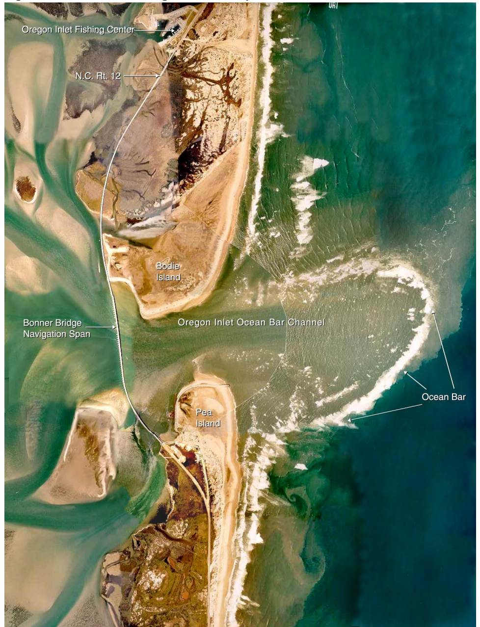
Figure 2: Aerial View of Oregon Inlet on September 18, 2001
