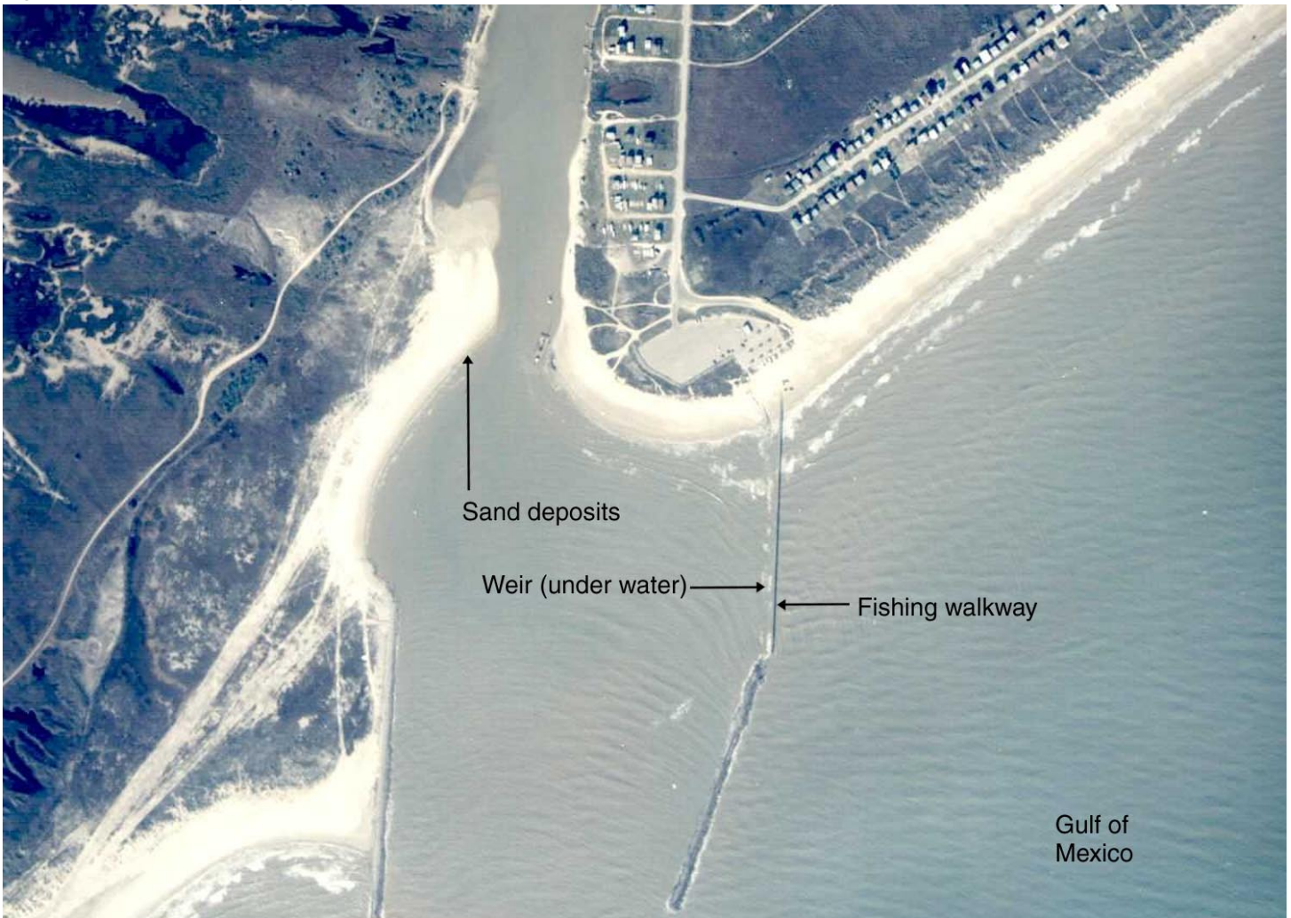
Figure 6: The Dual Jetty Project at Colorado River Inlet, Texas
