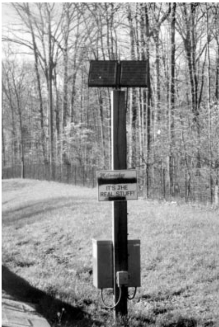
Traffic monitoring station
