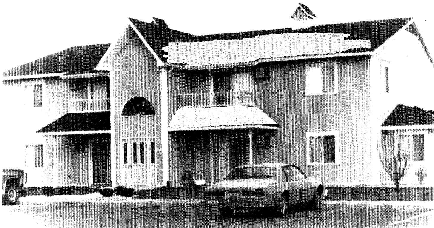
These apartments had sliding glass doors, balconies, and gutters and downspouts.
