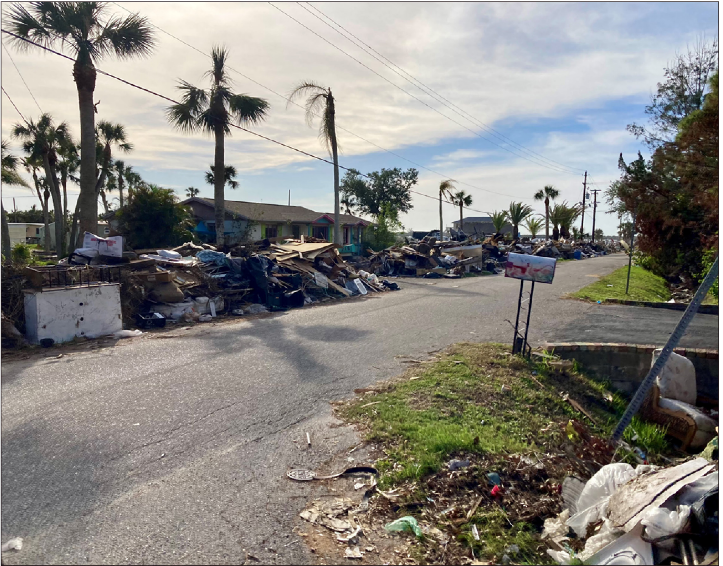
Figure 1: Debris from Damaged Homes Following Hurricanes Helene and Milton, 2024, Florida
