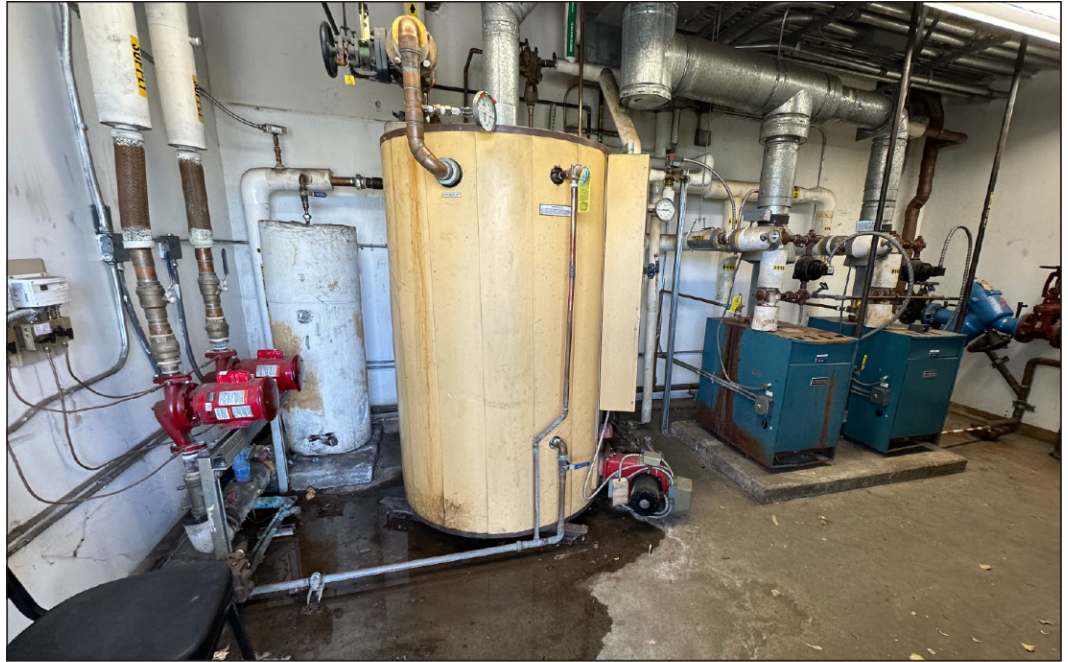
Figure 8: Example of Coast Guard Maintenance Project
