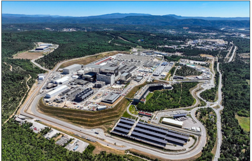
Figure 1: View of ITER Site, as of June 2024
