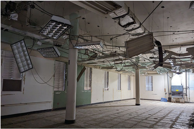
Room damaged by the hurricane in a facility that continues to support the Reserve Officers' Training Corps.
