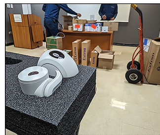
Digital infrastructure being installed into classroom
