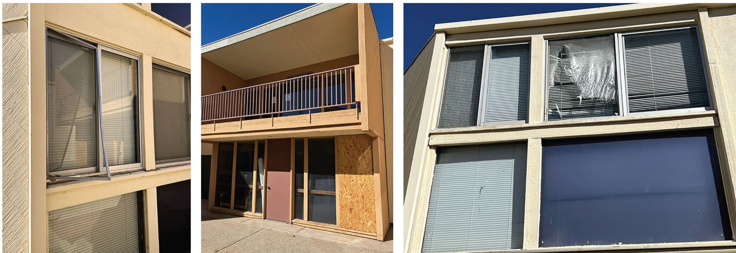
Figure 3: Example of Vacant Facility to Be Demolished on an HSI Campus
