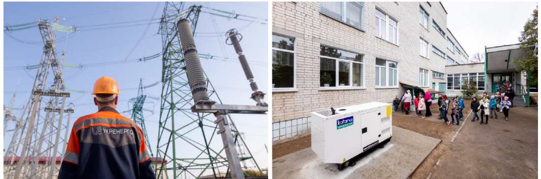
Figure 4: Modern Energy Services Assistance Included Activities to Support Ukraine's Energy Infrastructure and Generators
