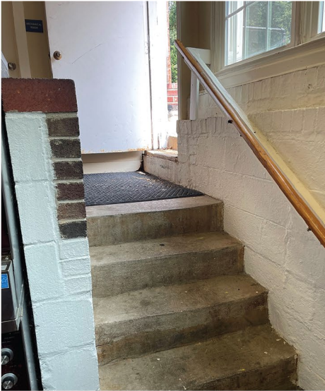
Stairs leading to multipurpose room
