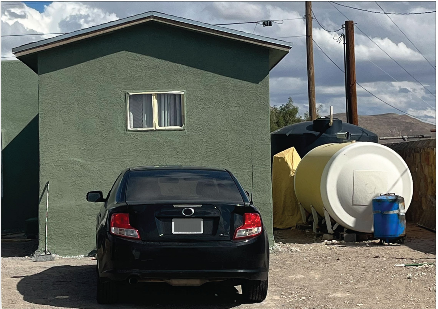
Figure 6: Cistern at a Home in a Texas Colonia
