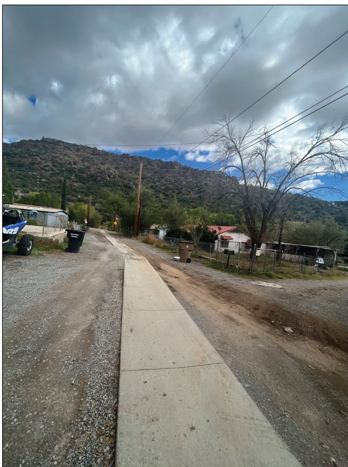
Drainage infrastructure funded by the CDBG colonias set-aside in an Arizona colonia.
