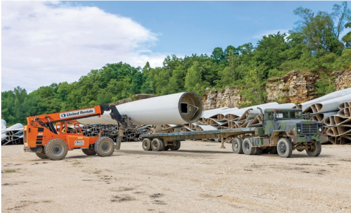
Figure 6: Partially disassembled turbine blades for recycling
