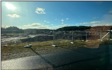
Kodiak Family Housing construction site.
