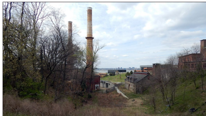
Coal combustion residue in a field at the St. Elizabeths campus in Washington, D.C. possibly originated from past use of the coal-fired power plants (pictured) and will be addressed in later re-development.
