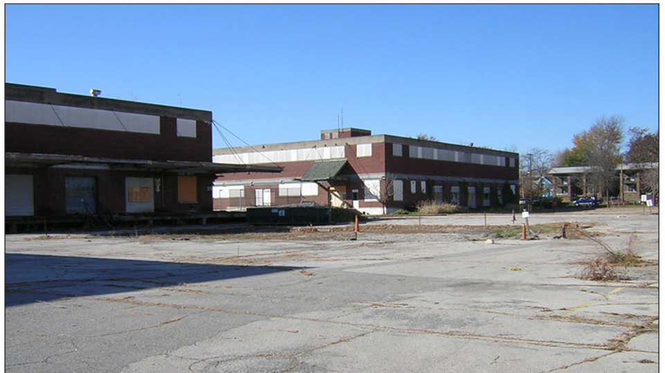
Figure 12: Former Hardesty Federal Complex, Kansas City, MO
