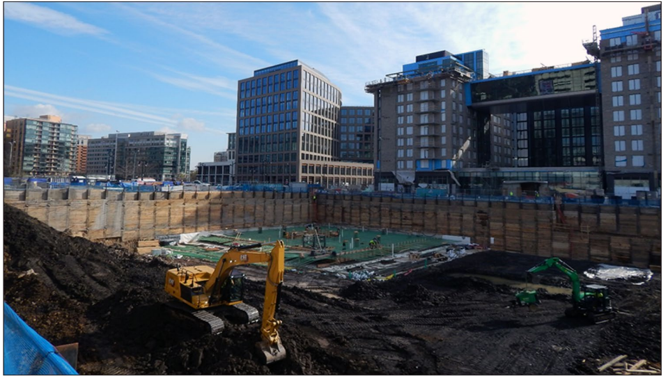
Figure 5: Cleanup of Previously Unknown Contaminated Soil Discovered during the Redevelopment of Southeast Federal Center, Washington, D.C.
