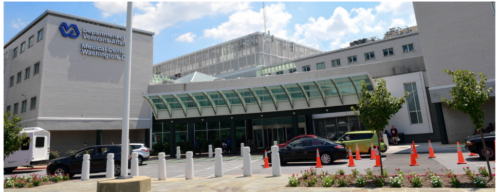
Source: GAO photo. | GAO-23-106765
