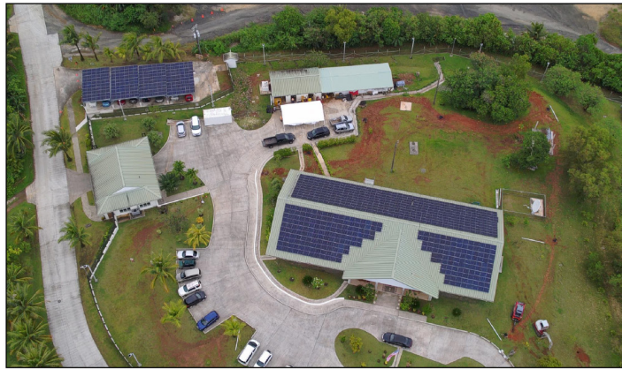
Koror, Palau, built in 2009, photovoltaic array installed in 2022.
