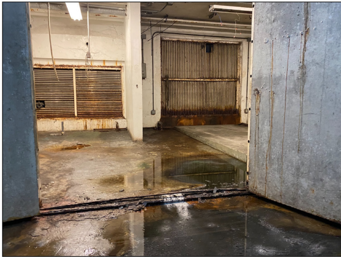
Chancery basement, subject to flooding, formerly housed generators.
