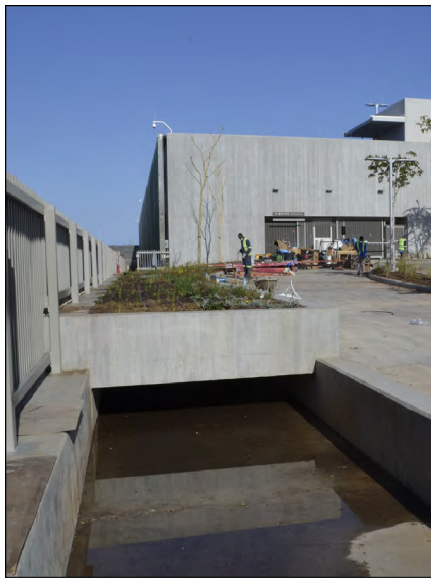
Storm water retention basins.
