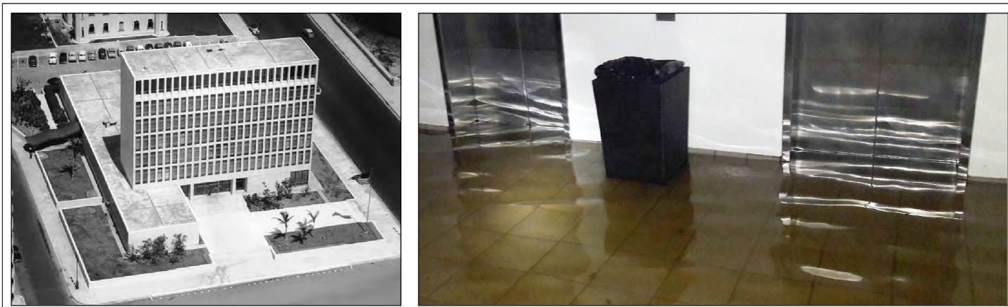
Figure 1: U.S. Embassy Havana, Cuba as Built in the 1950s (left), and Flooding within the Elevator Lobby from Hurricane Irma in 2017 (right)
