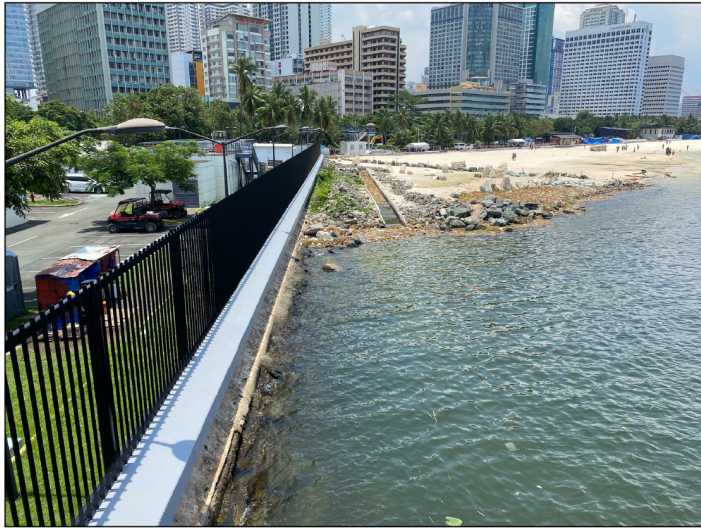
Manila Bay sea wall and stormwater outlet.
