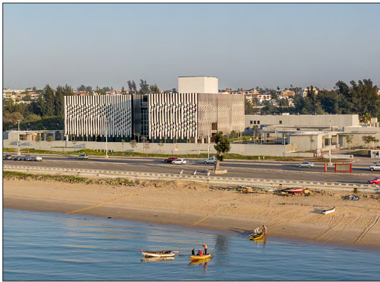
Exterior facade to reduce building heat gain.
