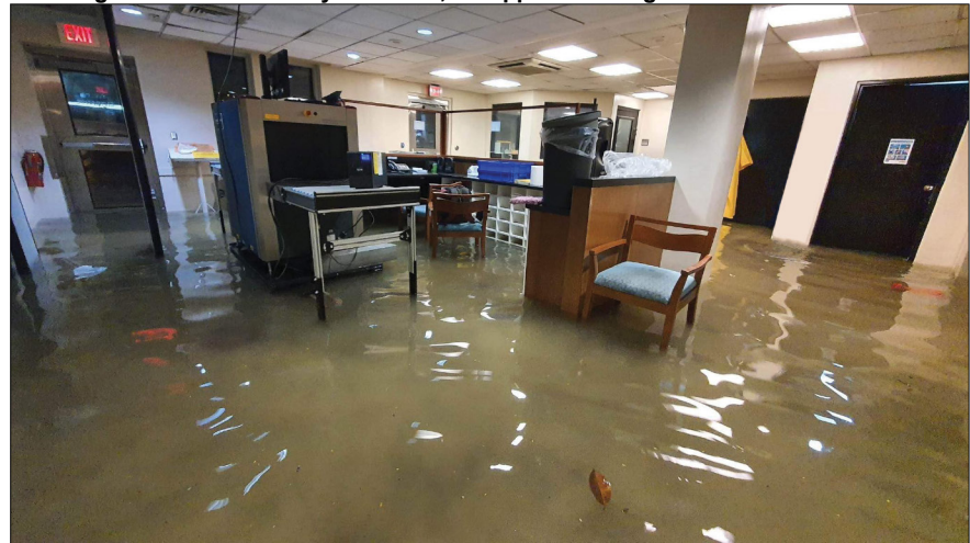
Flooding of the US. Embassy in Manila, Philippines in August 2022
