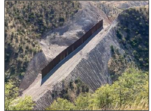
Erosion below the site of a cleared construction staging area (left); erosion below an area where only several border barrier panels were installed as of January 2021 (right).
