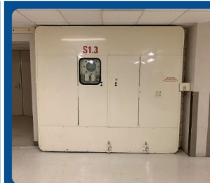
Watertight enclosure to prevent floodwater damage
