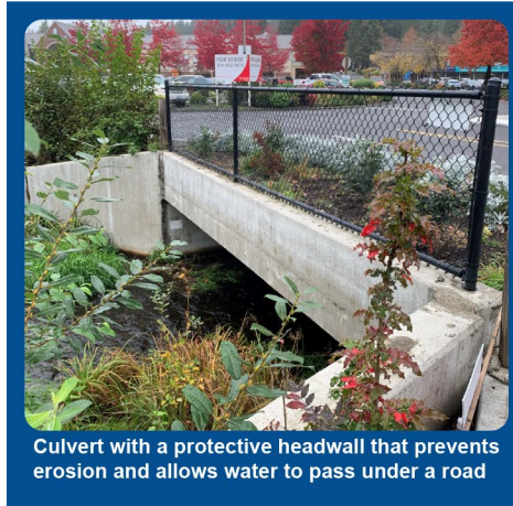
Figure 2: Examples of Hazard Mitigation Projects
