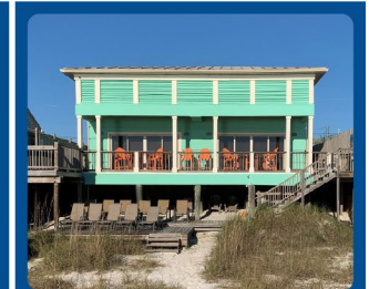
Structure elevation to mitigate flood damage
