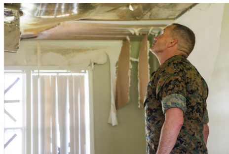
Marine Corps Base Camp Lejeune, North Carolina (2018) Damage from Hurricane Florence a
