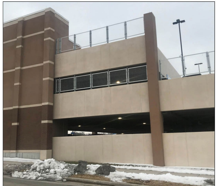
Heightened barriers at a parking garage to prevent efforts to jump off the structure.
