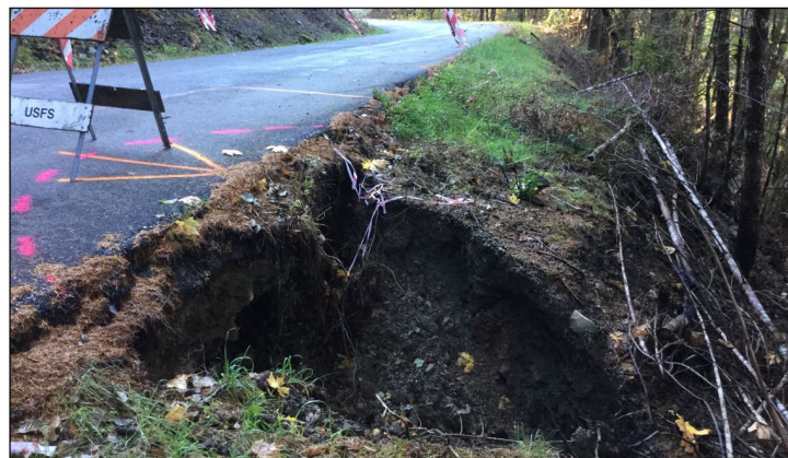
Figure 9: Culvert and Road Damaged by Erosion following the Chetco Bar Fire, October 2017
