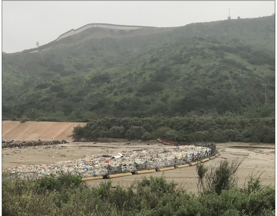
Figure 9: Trash Boom in a Canyon Collector in the Tijuana River Valley Watershed in California
