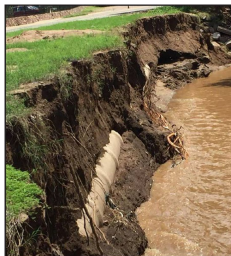
3rd Section Total length = approximately 7 miles A pipeline adjacent or underneath the Nogales Wash.
