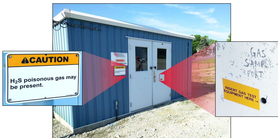
Figure 3: Hydrogen Sulfide Warning at a Natural Gas Storage Site
