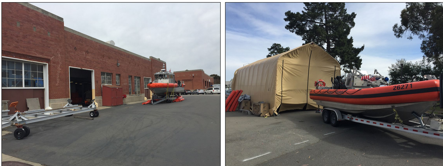
Figure 3: Coast Guard Maintenance Facilities Requiring Refurbishment Because They Cannot Accommodate Newer, Taller Boats
