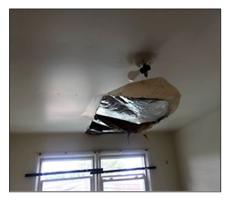
Ceiling damage from a roof leak
