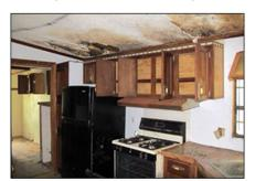
Mold and ceiling damage in kitchen
