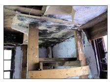
Mold damage in basement
