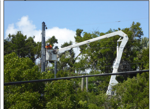
Wooden utility poles for electricity distribution are being replaced by composite fiberglass poles that can withstand 200 mile per hour winds.
