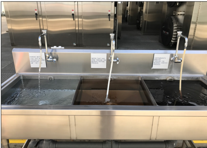
Photo on the left shows reused water at different points in the treatment process, and photo on the right shows reverse osmosis equipment at Orange County’s Groundwater Replenishment System, as of April 2018. The Groundwater Replenishment System was funded in part by the Bureau of Reclamation’s Title XVI Water Reclamation and Reuse Program.
