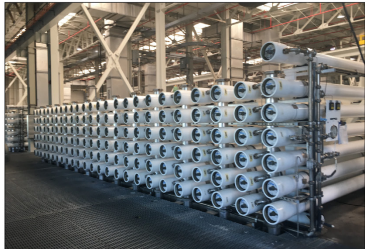
Photo on the left shows reused water at different points in the treatment process, and photo on the right shows reverse osmosis equipment at Orange County’s Groundwater Replenishment System, as of April 2018. The Groundwater Replenishment System was funded in part by the Bureau of Reclamation’s Title XVI Water Reclamation and Reuse Program.
