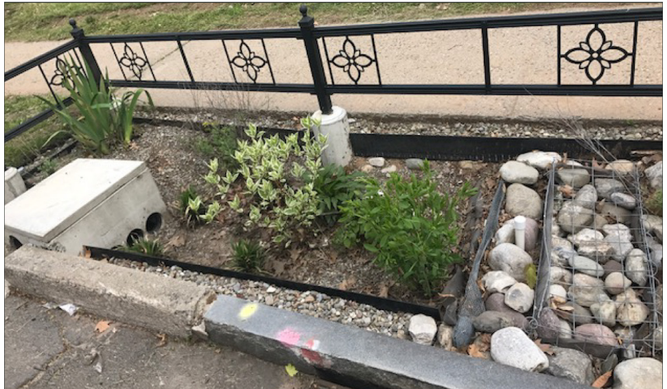
Figure 3: Bioswale in the Long Island Sound Watershed Used to Slow and Filter Pollutants from Stormwater Runoff
