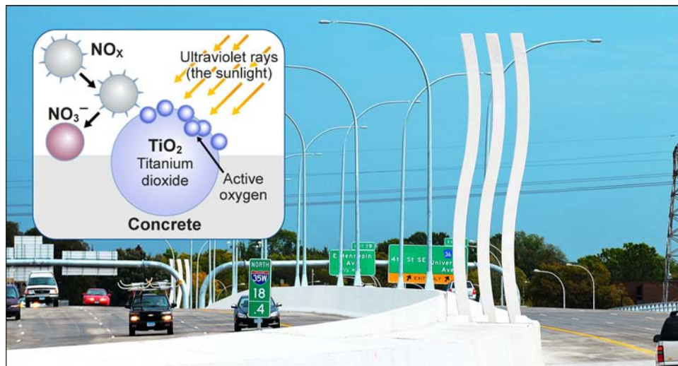
Figure 21: Removal of Harmful Pollutants by Nanotechnology-Based Concrete in Sculpture
