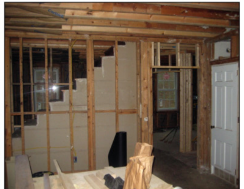
Building under renovation.
