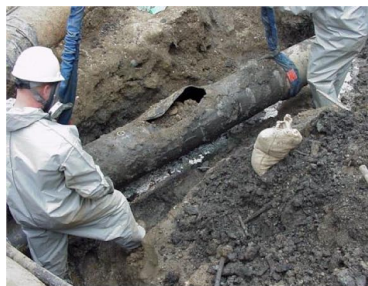
Source: National Transportation Safety Board.
