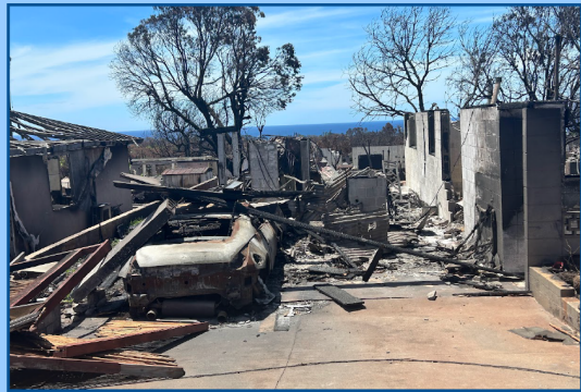
Figure 8: Wildfire Debris Removal in Lahaina, Hawaii
