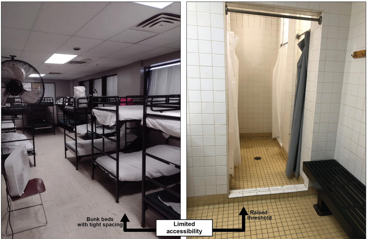
Figure 9: Example of a Shelter Room with Bunk Beds and Shower Area with a Raised Threshold
