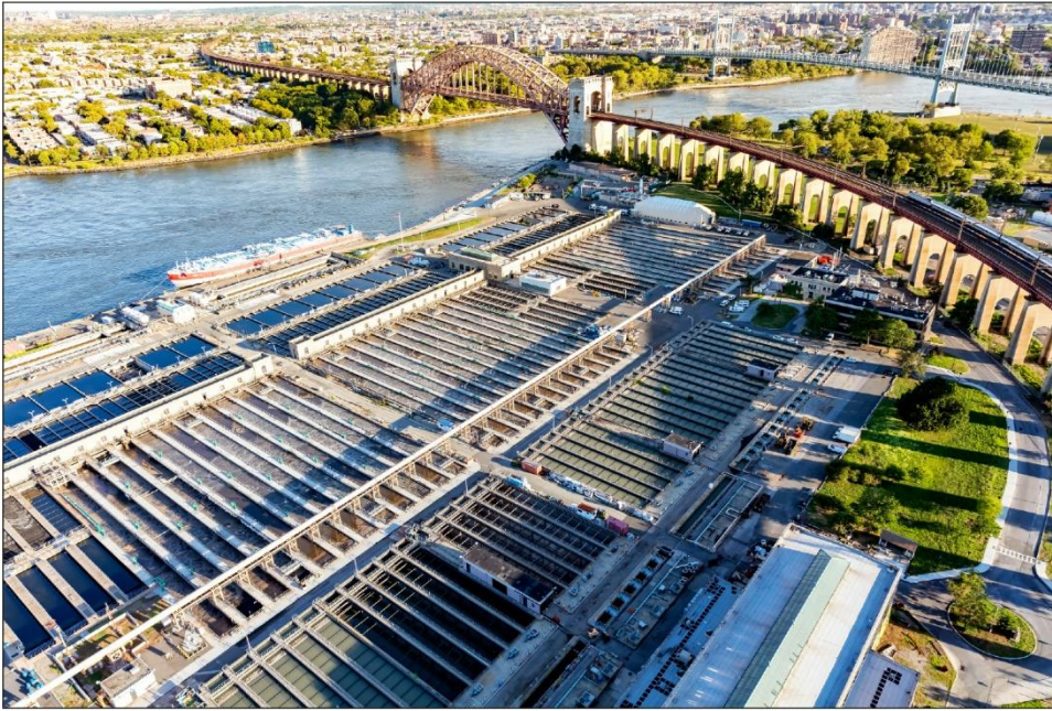
Aerial view of Wards Island Wastewater Treatment Plant in New York City.
