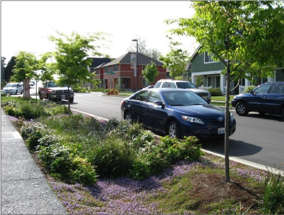
Figure 4: Example of a Bioswale Used for Stormwater Management
