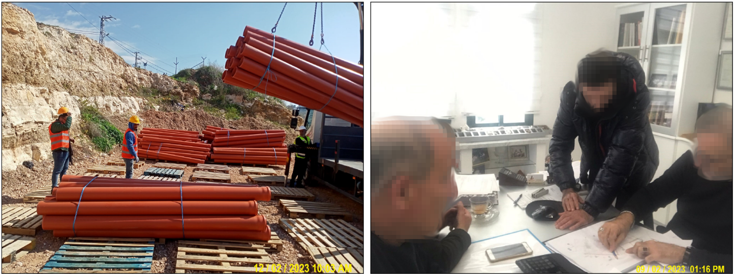
Figure 5: Workers at a Wastewater Collection System Improvements Project Funded by USAID
