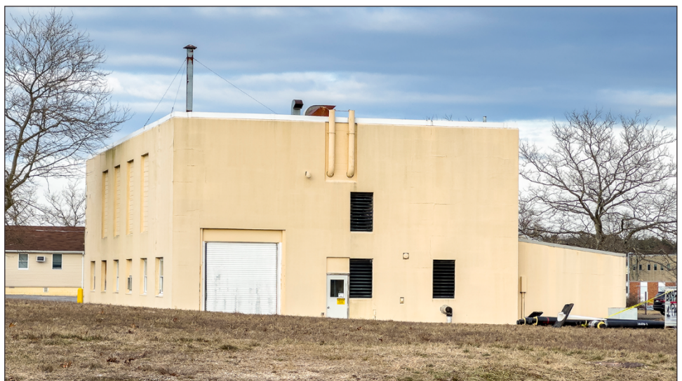
Figure 7: Deliberately Deferred Maintenance and Repair: Retired Brookhaven National Laboratory Steam Plant
