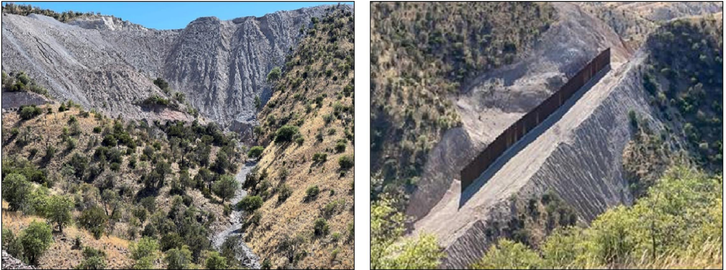
Figure 2: Erosion on the Coronado National Forest in Arizona (May 2022)
