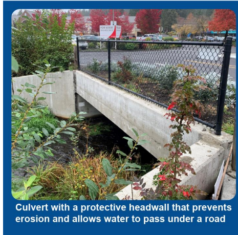
Figure 2: Examples of Hazard Mitigation Projects
