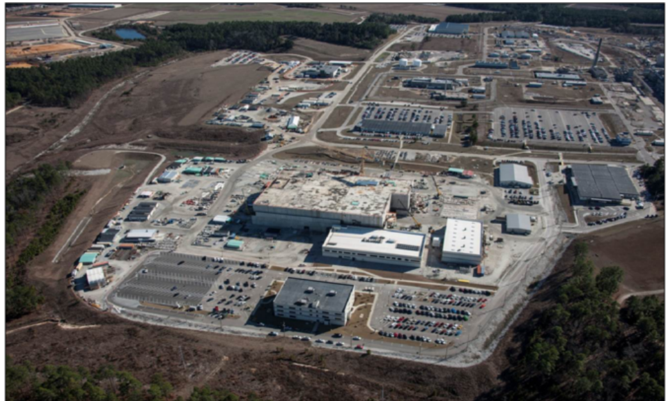
Figure 14: Partially Completed NNSA Construction Project Cancelled in 2018 Following Adoption of New Project Management Practices
