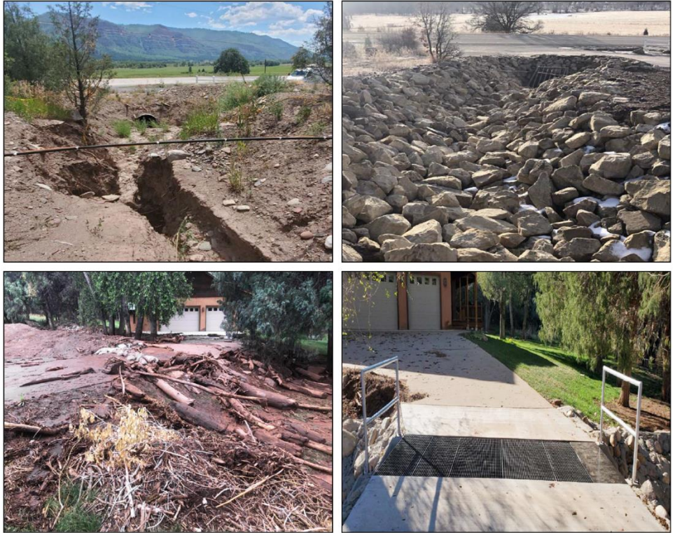
Figure 2: Post-Wildfire Flood Damage and Emergency Measures in Colorado
