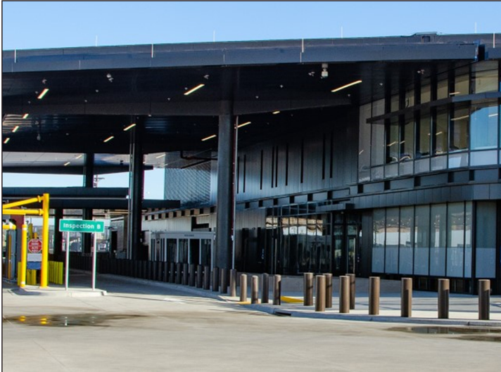
Figure 3. Department of Homeland Security's (DHS) Calexico, CA, Land Port of Entry Project
