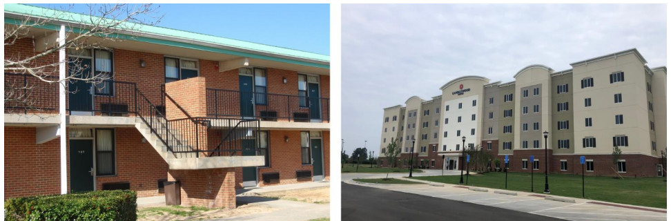
Figure 14: The Army Replaced Lodging at Fort Gordon, GA, with a Candlewood Suites Hotel in 2020 as Part of the Privatized Army Lodging Program
