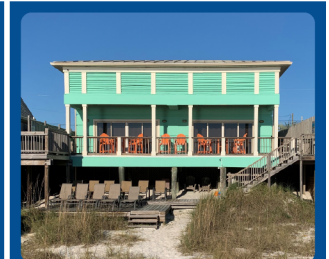
Structure elevation to mitigate flood damage
