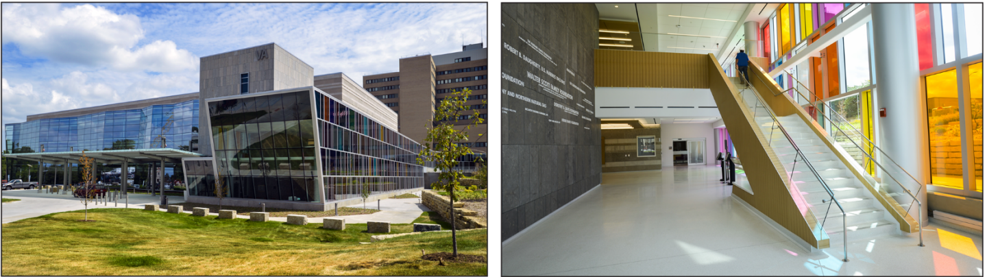
Figure 2: Department of Veterans Affairs’ (VA) Ambulatory Care Center in Omaha, NE—Exterior and Interior Views
