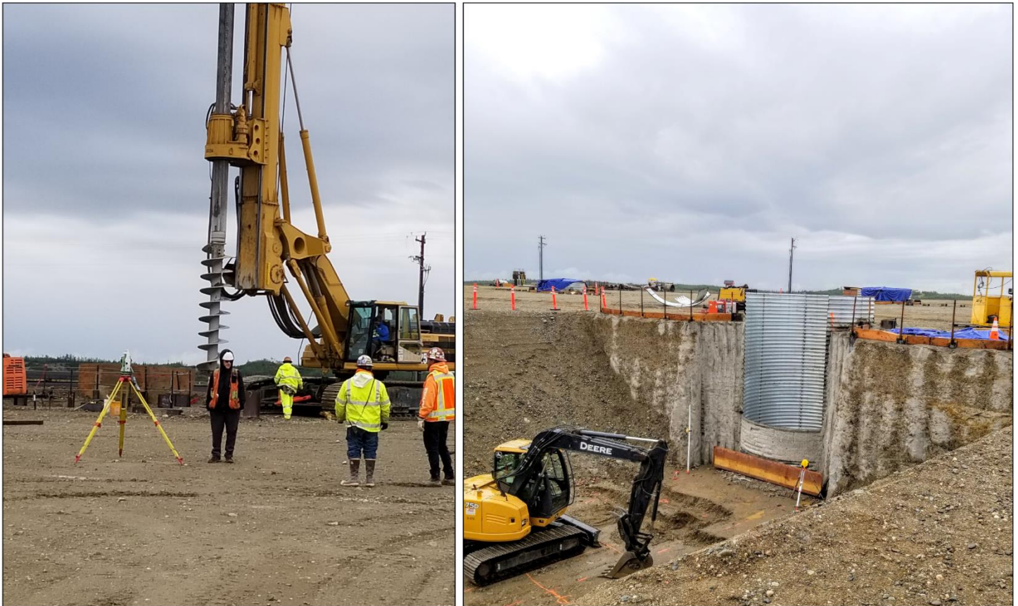
Figure 12: Ongoing Construction of Missile Field 4 at Fort Greely, Alaska (July 16, 2019)
