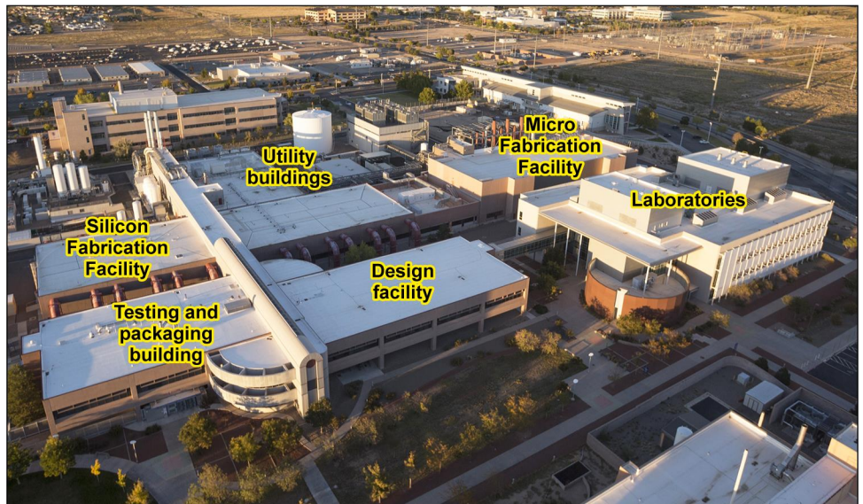
Figure 1: Aerial View of the Microsystems Engineering, Sciences and Applications Complex at Sandia National Laboratories
