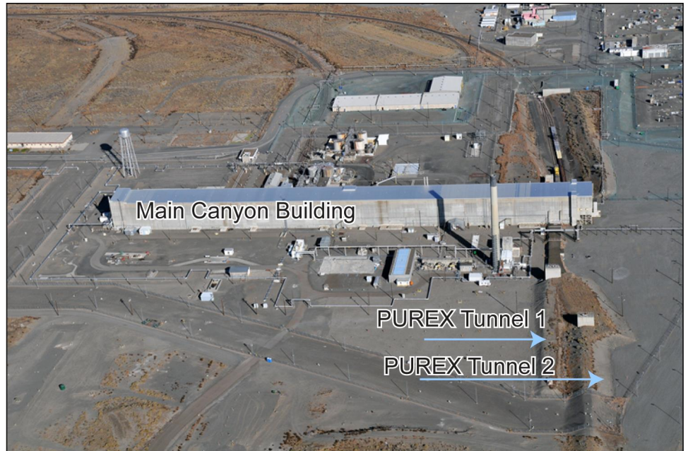
Figure 3: Main PUREX Plant and Auxiliary Facilities
