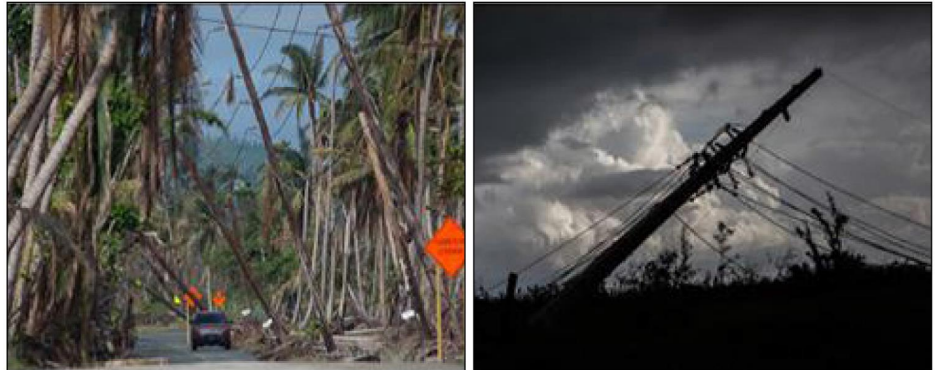
Damaged Power Lines in Puerto Rico in November 2017 after Hurricane Maria
