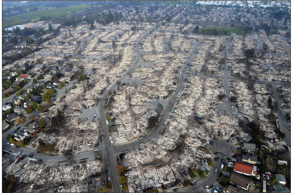
Figure 10: Aerial Photograph of Damage from Tubbs Fire, Santa Rosa, California, October 11, 2017
