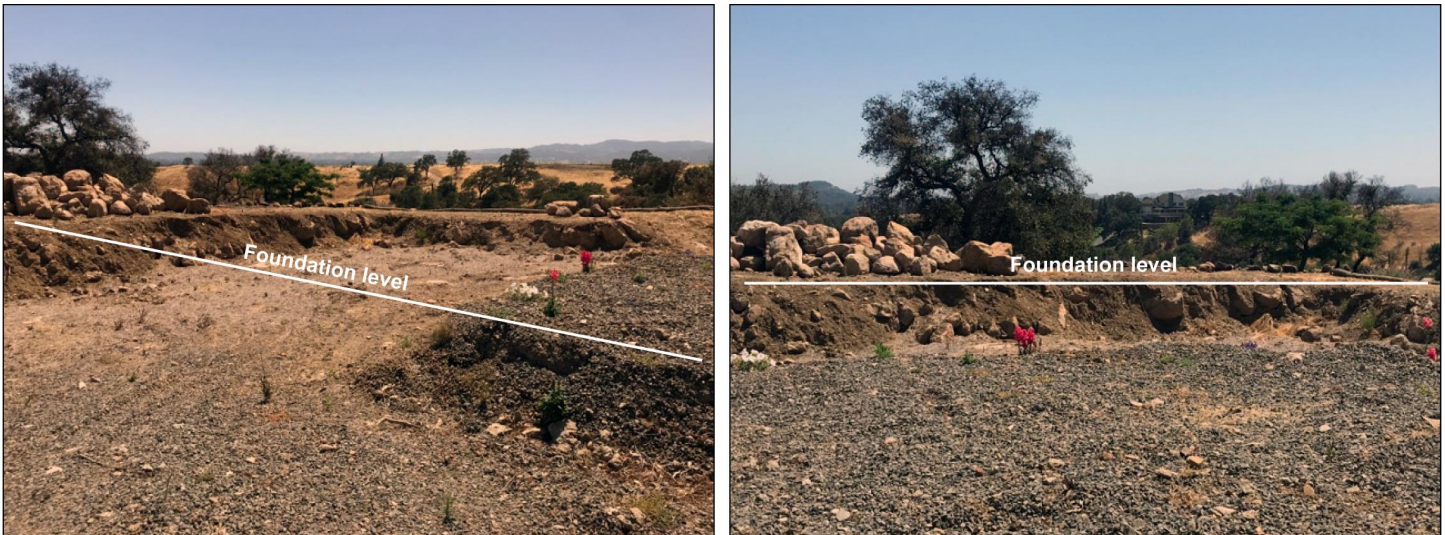
Figure 5: Excavated Residential Property Site, Napa, California
